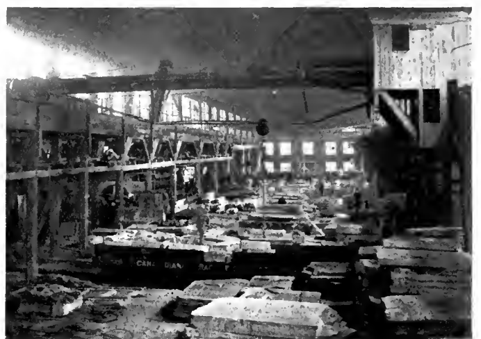
Interior of Lyall Mill, Wallace Sandstone Quarries Co.
